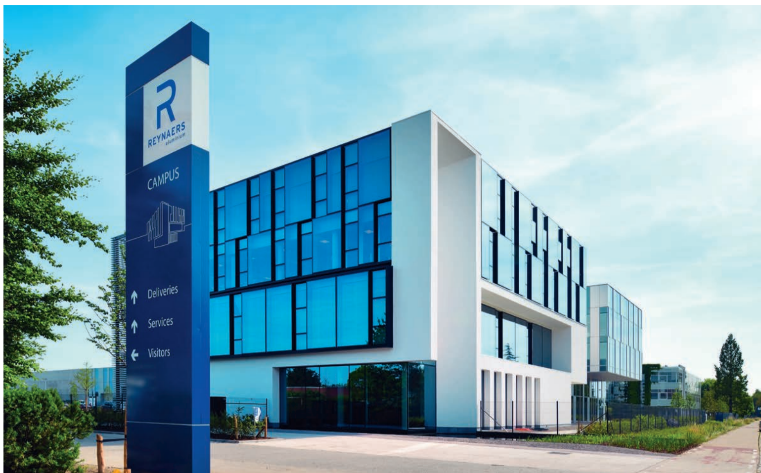
Headquarters of Reynaers Aluminium in the Belgian municipality of Duffel Image: Reynaers Aluminium
