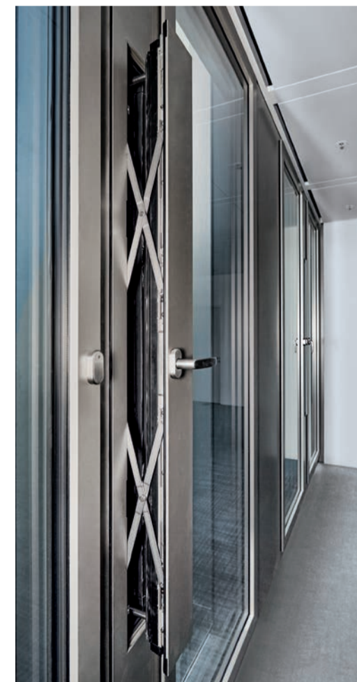
The ventilation flaps in the Marienurm were equipped with parallel projecting scissor stays from the Roto PS Aintree range.
