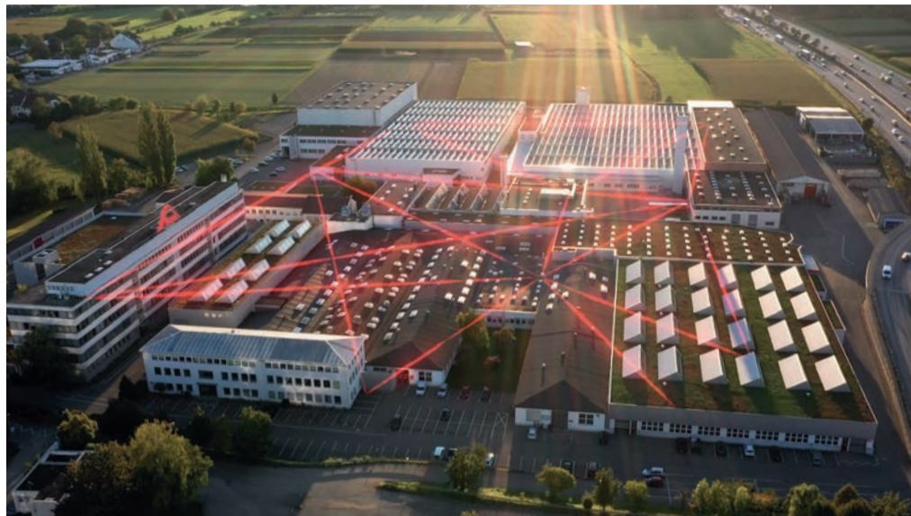
Many digitalisation projects are aimed at enabling machines, tools and vehicles in the 15 production plants of Roto FTT to optimise their performance autonomously.
