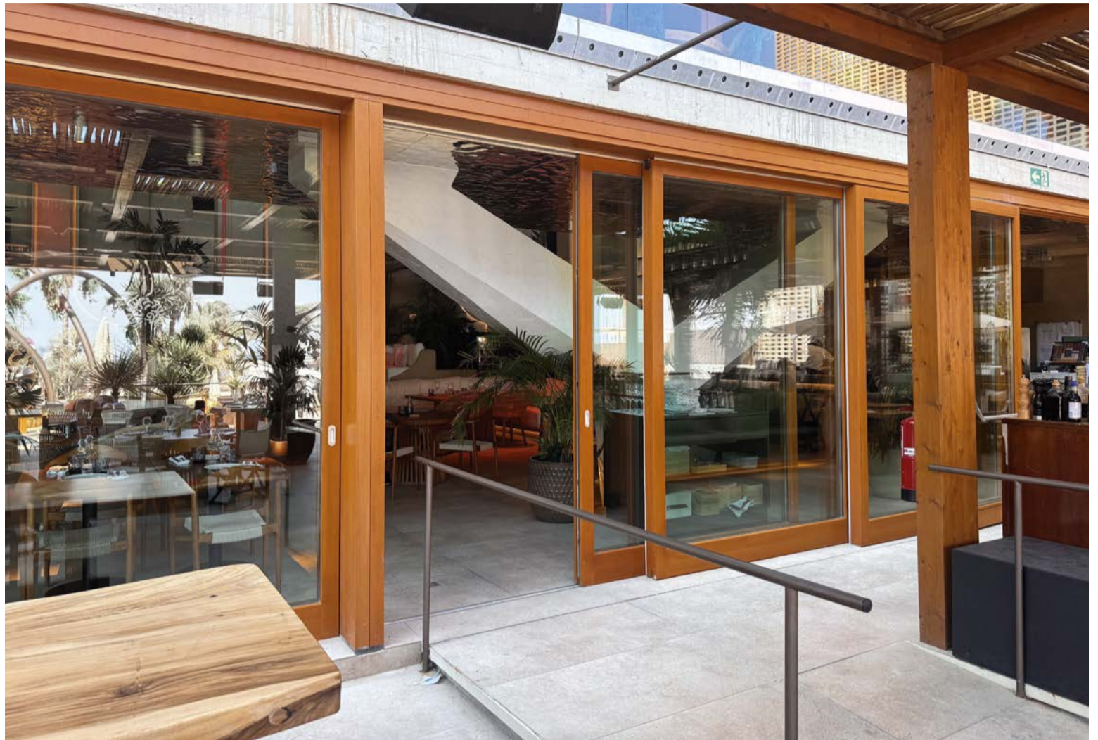
Deko Grup-35 produced around 150 fixed glazing units, Tilt&Turn windows and sliding elements from spruce timber for the building, which dates back to the 1970s. The ROI Plus 70.2 and 90.3 profile systems were used.
